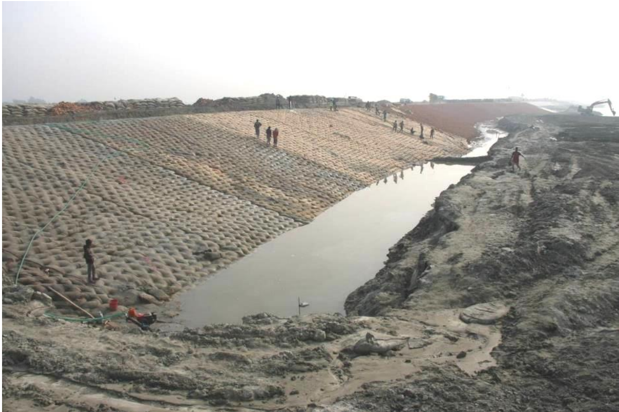
Figure 4-3. Installation of grout-filled jute mattress (Harirampur Feb 2019)
