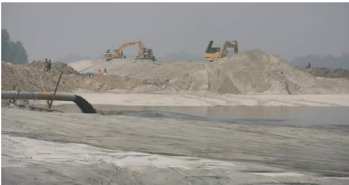
Figure 4-4. Embankment construction at JRB-1 with compacted dredged sand (Kaijuri,
