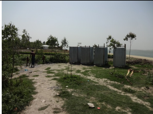
3. Toilets (4) in worker's camp (for about 350 workers).
