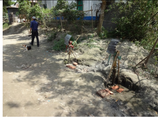
2. Two tubewells in worker's camp, one is operational.
