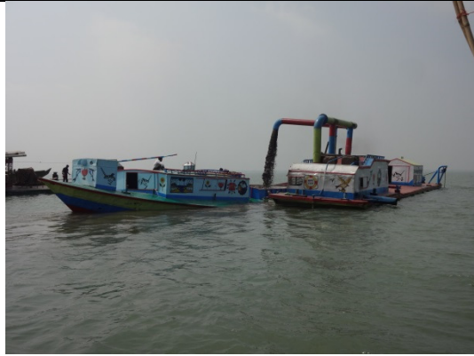
1. Sand mining from a dredger in the middle of Padma River
