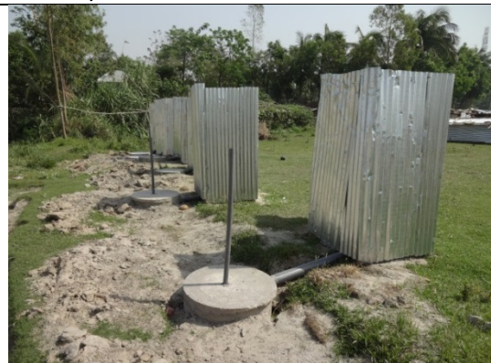
6. Toilets (6) for about 400 workers
