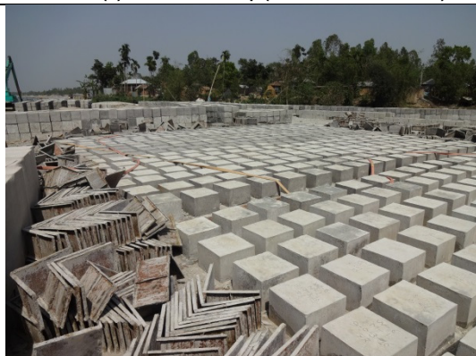
5. Site for making concrete blocks.
