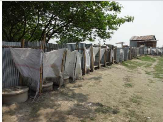
7. Toilet facilities for 1400 labourers
