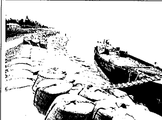
1. Riverbank protection by sandbags
