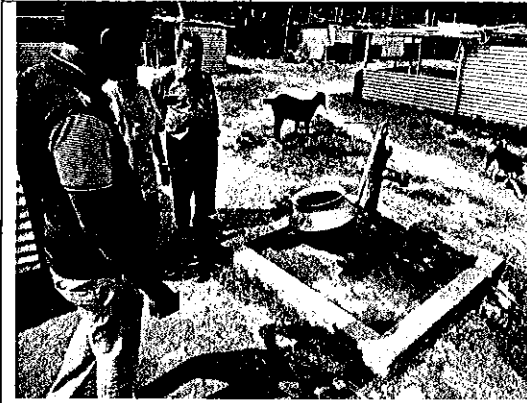
3. Concrete protection around tubewell in worker's camp
