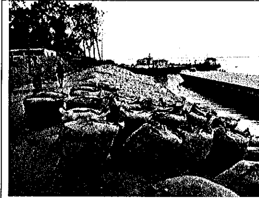
1. Riverbank protection with sandbags opposite the site office (viewed towards south)
