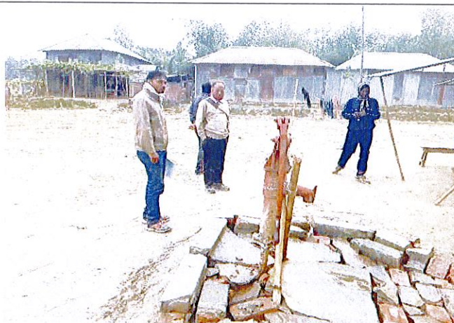
5. Broken protection of tube well
