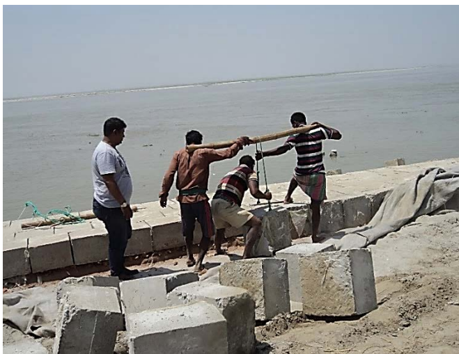
5. C.C block is placing with risk
