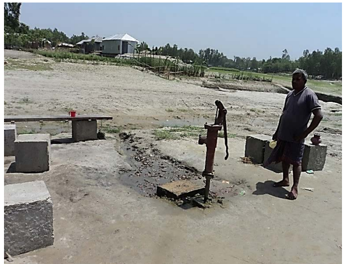
4. Tube well with no protection directly discharge in field
