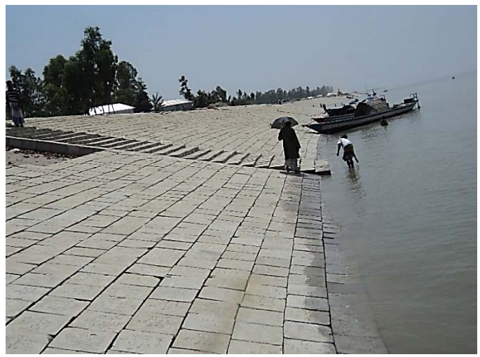
6. Completed bank protection work with stair.
