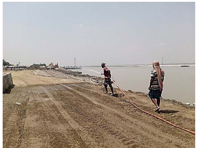
2. Water is being spraying on road for dust suppression
