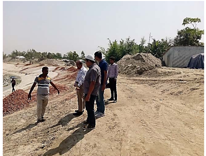
2. Slope is being built as per design
