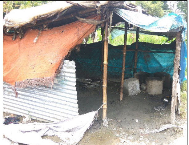
2. Kitchen with enclosure and roof
