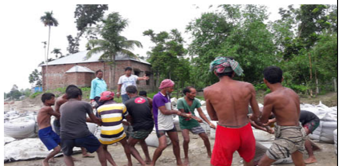
6 Geo-textile bags are being placed to fight with Erosion
