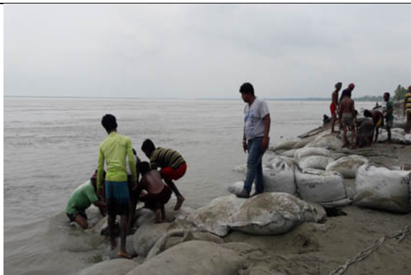
5 C.C block is placing with risk
