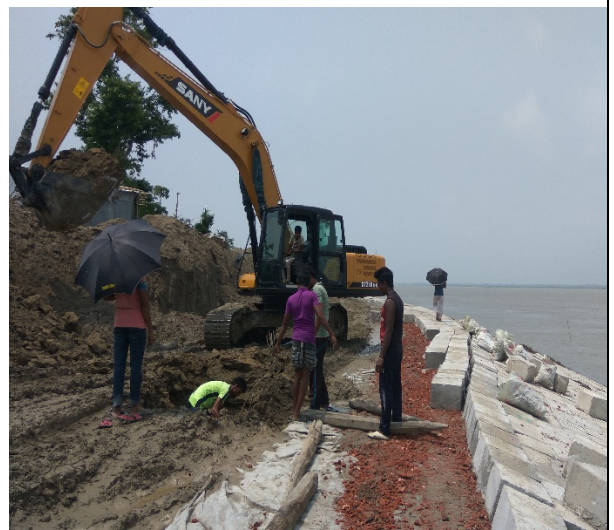
6. The slope building work
