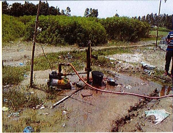
2. Tube well without protection
