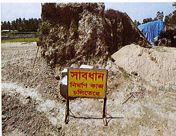
5. Safety warning sign displayed at site
