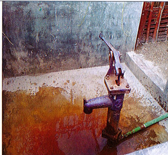
3. Tube well without protection
