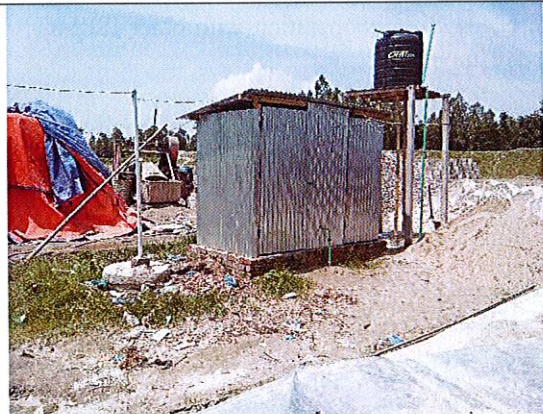
3. Sanitary toilet with sock pit
