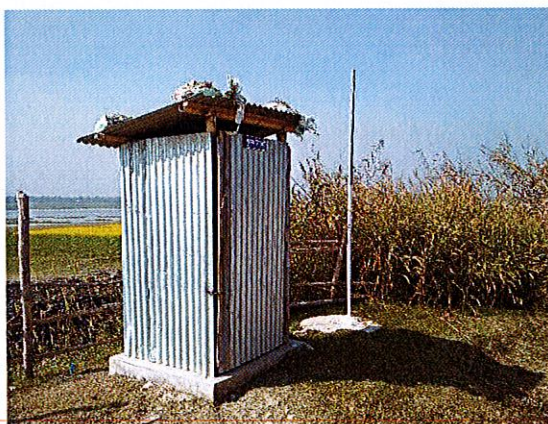
5. Sanitary toilet with sock pit
