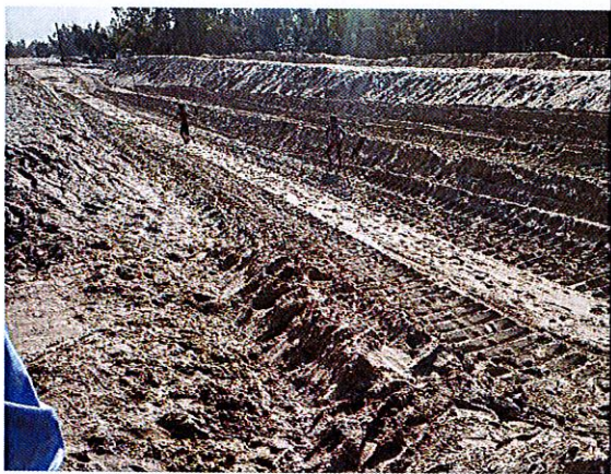
5. Construction of Embankment
