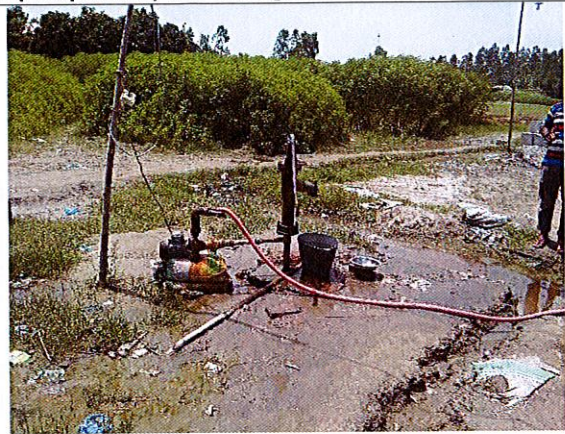
2. Tube well without protection
