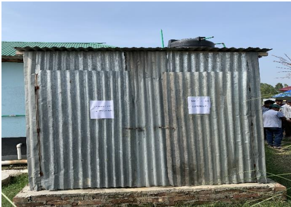
3. Sanitary toilet with sock pit
