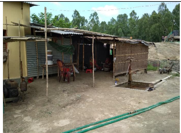
2. Tube well with protected base
