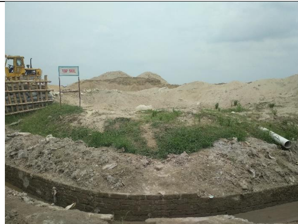
4. Preservation of Top soil
