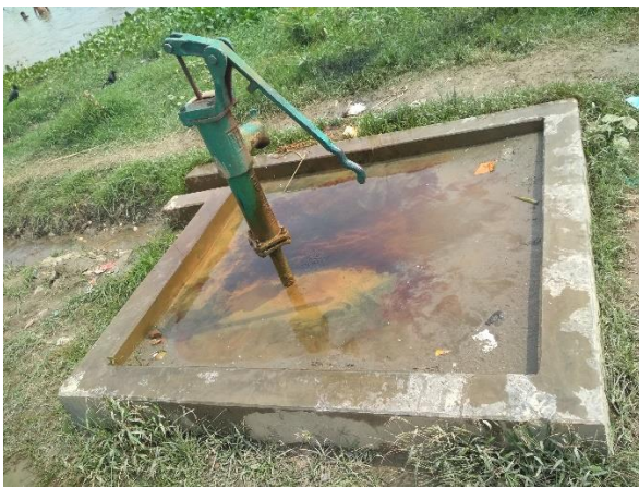
5. Tube well with protected base
