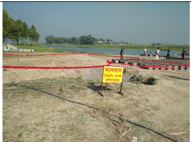
2. Safety warning sign at working site
