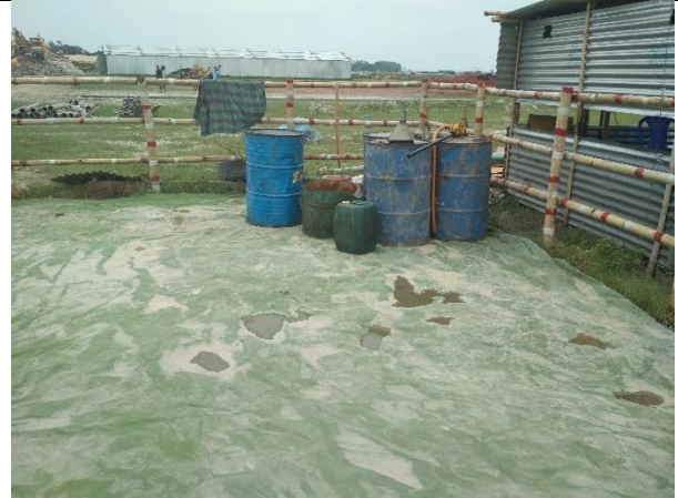
2. Fuel & lubricants are stored under open sky
