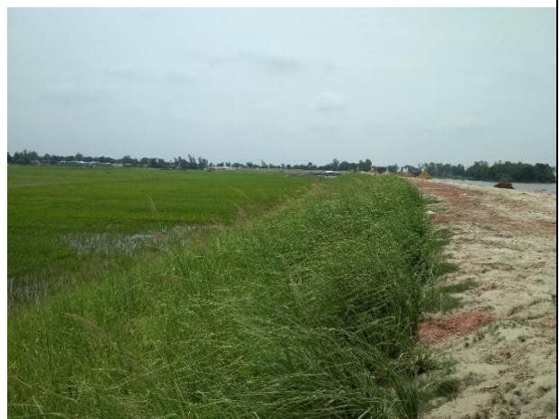
6. Vativer grass grown at the embankment
