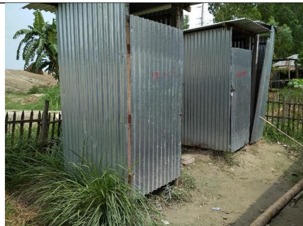
4. Sanitary toilet with sock pit
