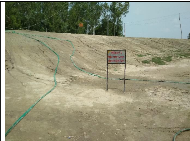
1. Safety signboard at the working site
