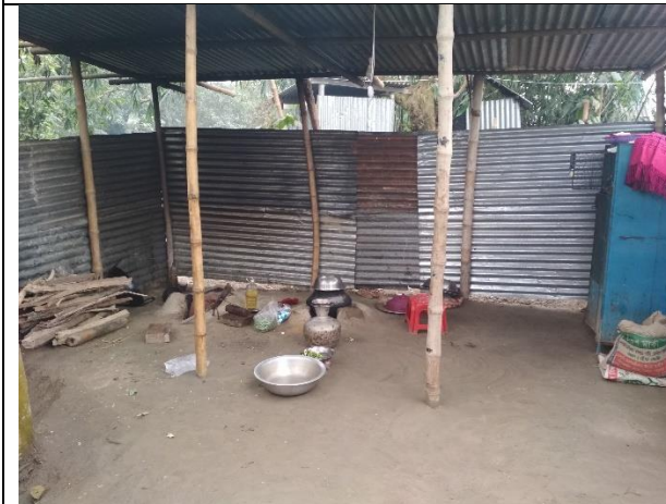
3. Kitchen with C.I sheet roofing and enclosure
