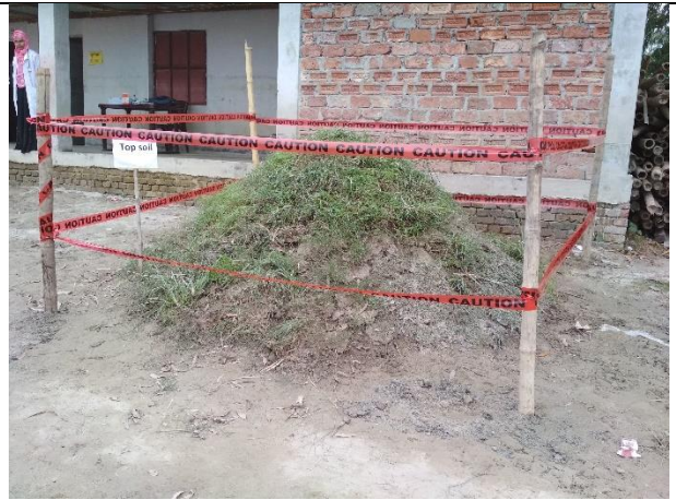
2. Preservation of Top soil
