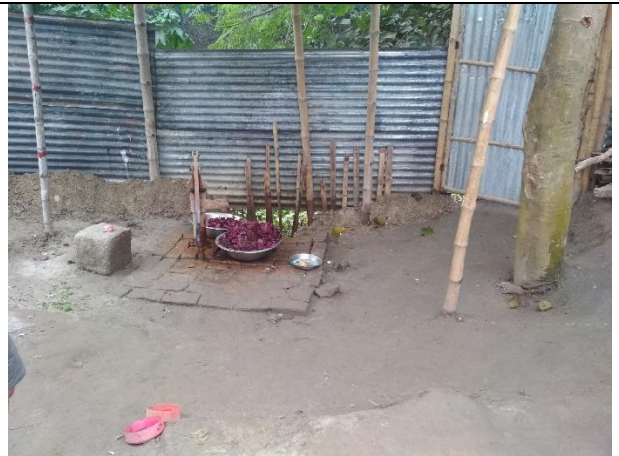
2. Tube well with protected base
