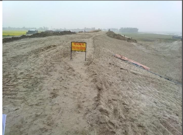
4. Safety warning signboard displayed at site
