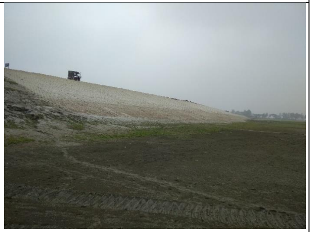
6. Completed Embankment with grout filled jute mattress
