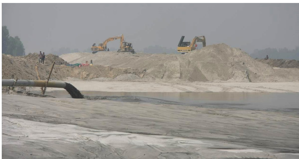
Figure 2-7 Embankment construction at JRB-1 with compacted dredged sand (Kaijuri, Feb 2019)
