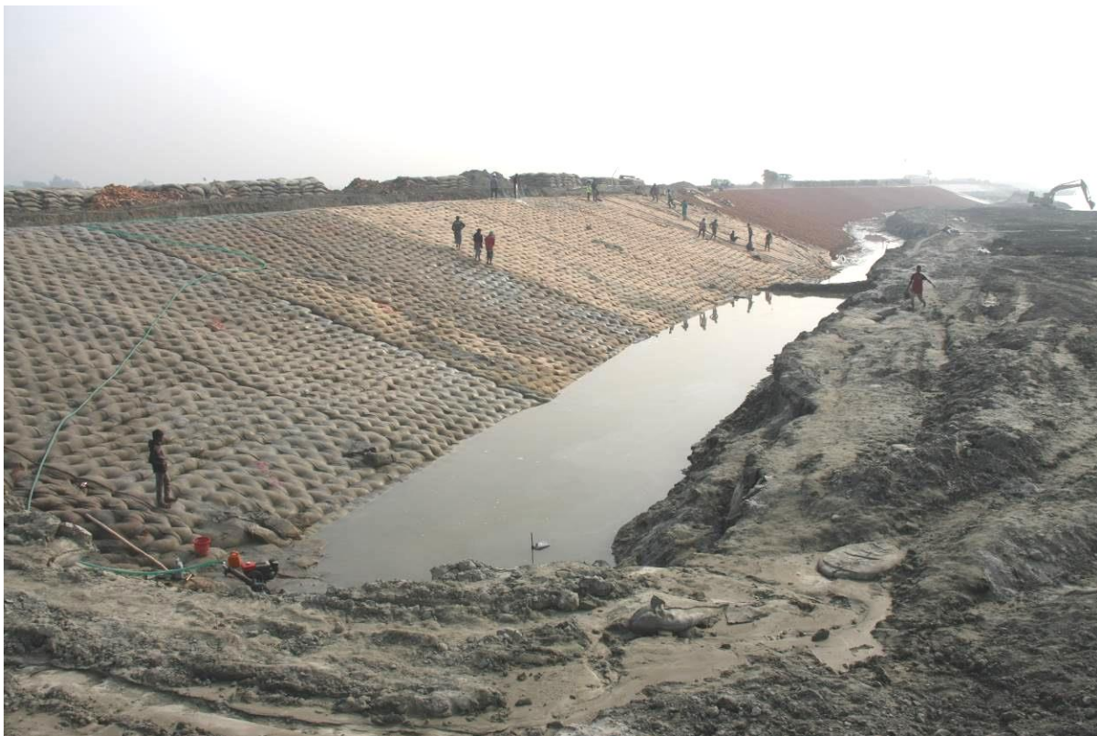
Figure 2-6 Installation of grout-filled jute mattress (Harirampur Feb 2019)
