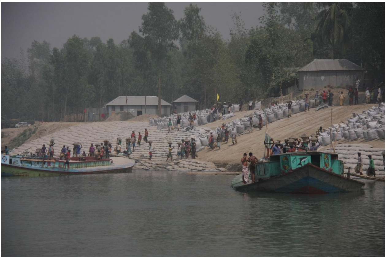
Placement of first temporary wave protection, 5 March 2016
