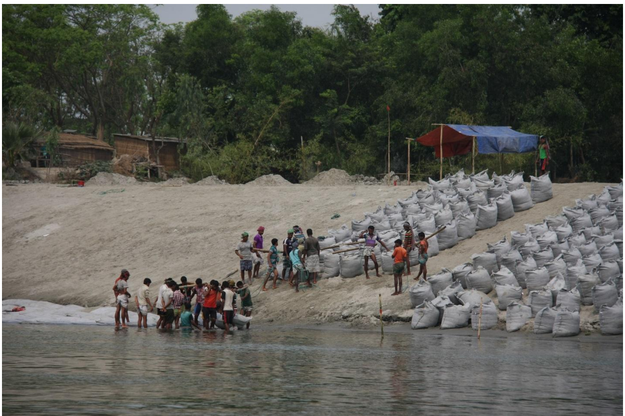
Wave protection work ongoing, 14 March 2016
