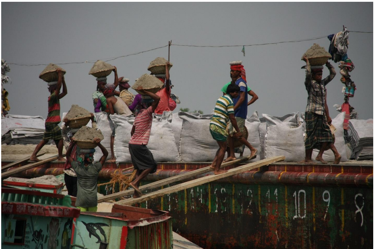
Filling of geobags for next dumping sequence, 14 March 2016
