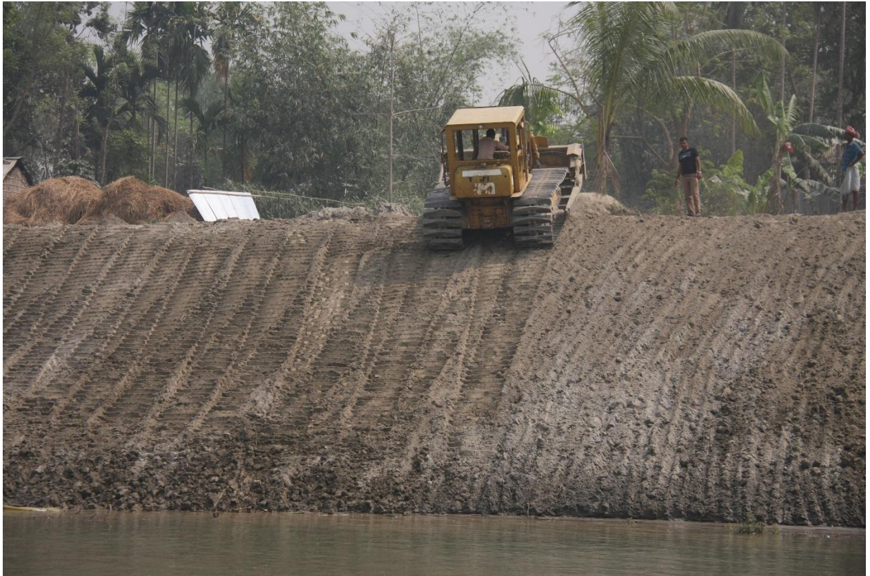
Preparation of slope for temporary wave protection in Chauhali, 5 March 2016
