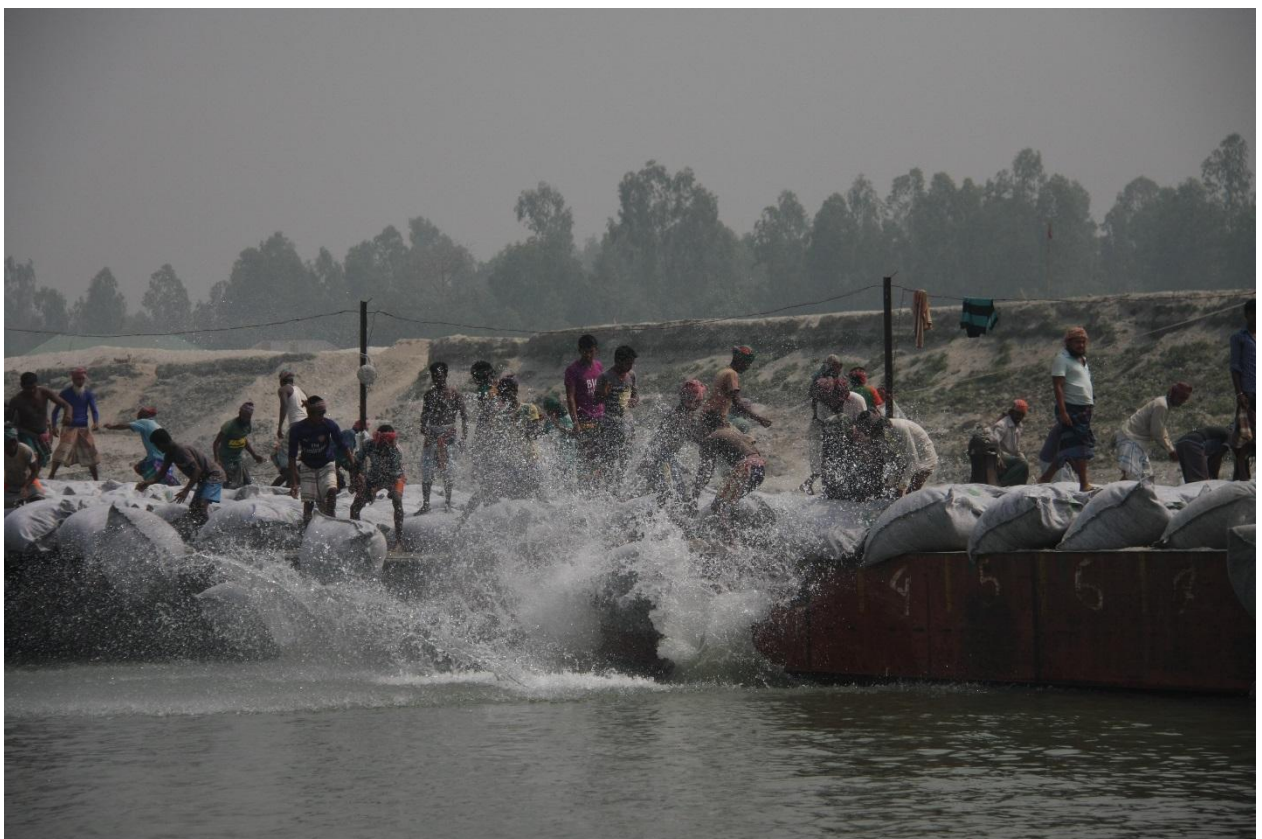
Geotextile bag dumping in Chauhali, 5 March 2016
