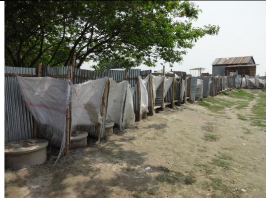
7. Toilet facilities for 1400 labourers
