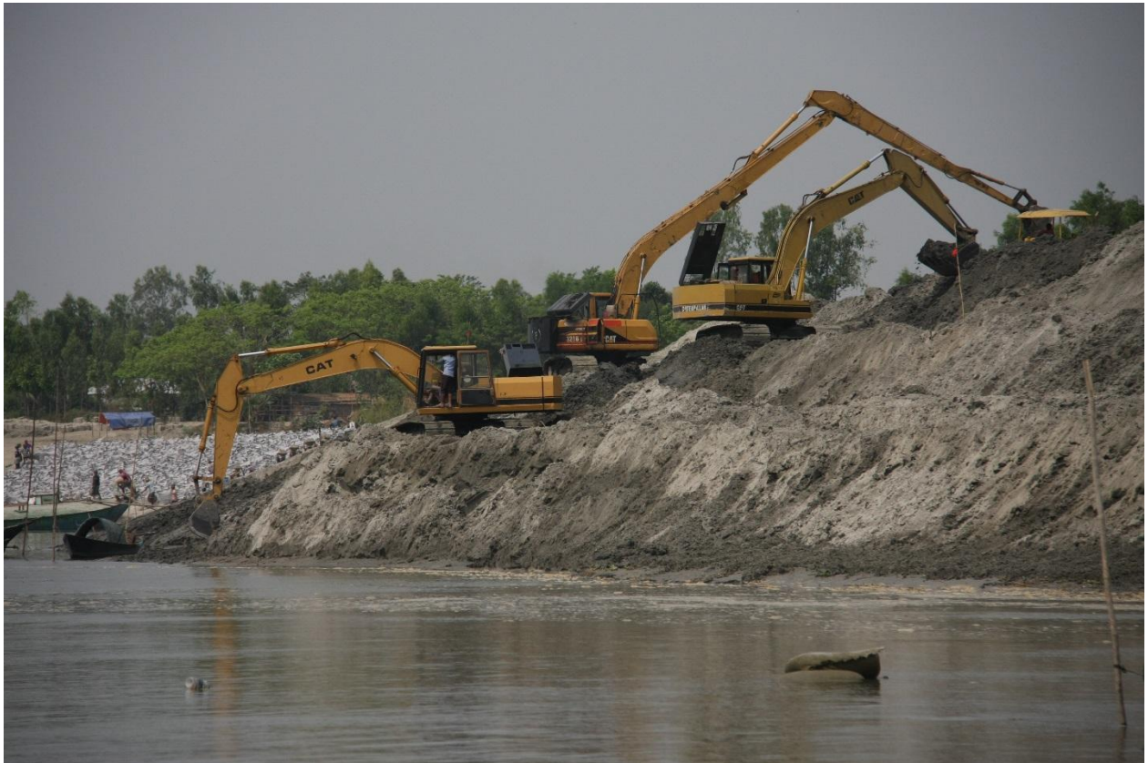
Preparation of slope for wave protection on 14 March 2016
