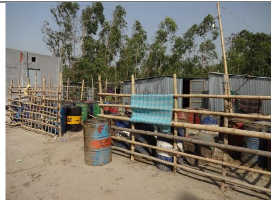
16. Fencing of fuel & lubricant storage
