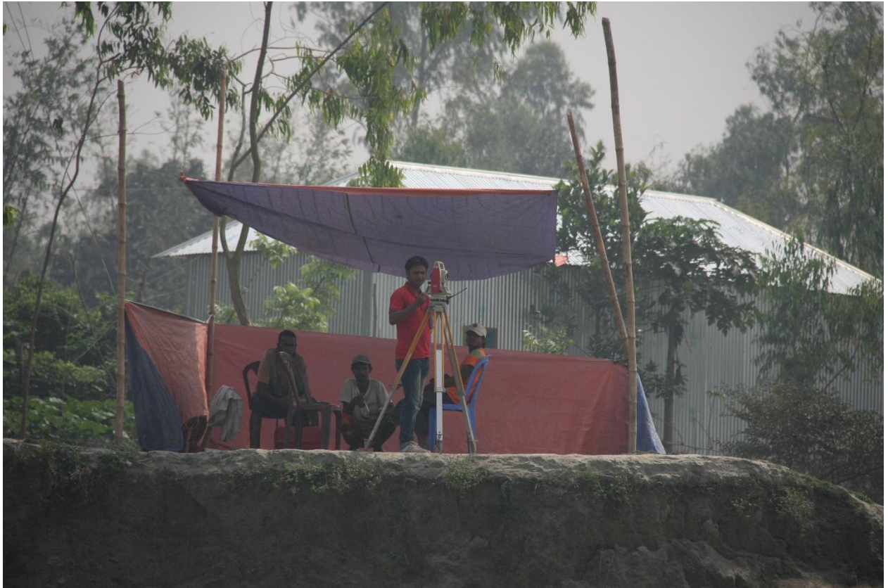
Positioning of barges at Chauhali, 5 march 2016
