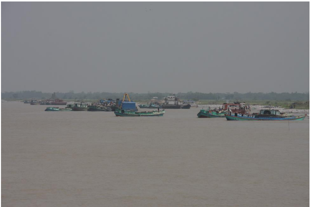
Construction at Harirampur with multiple sets of dumping barges, 26 May 2016
