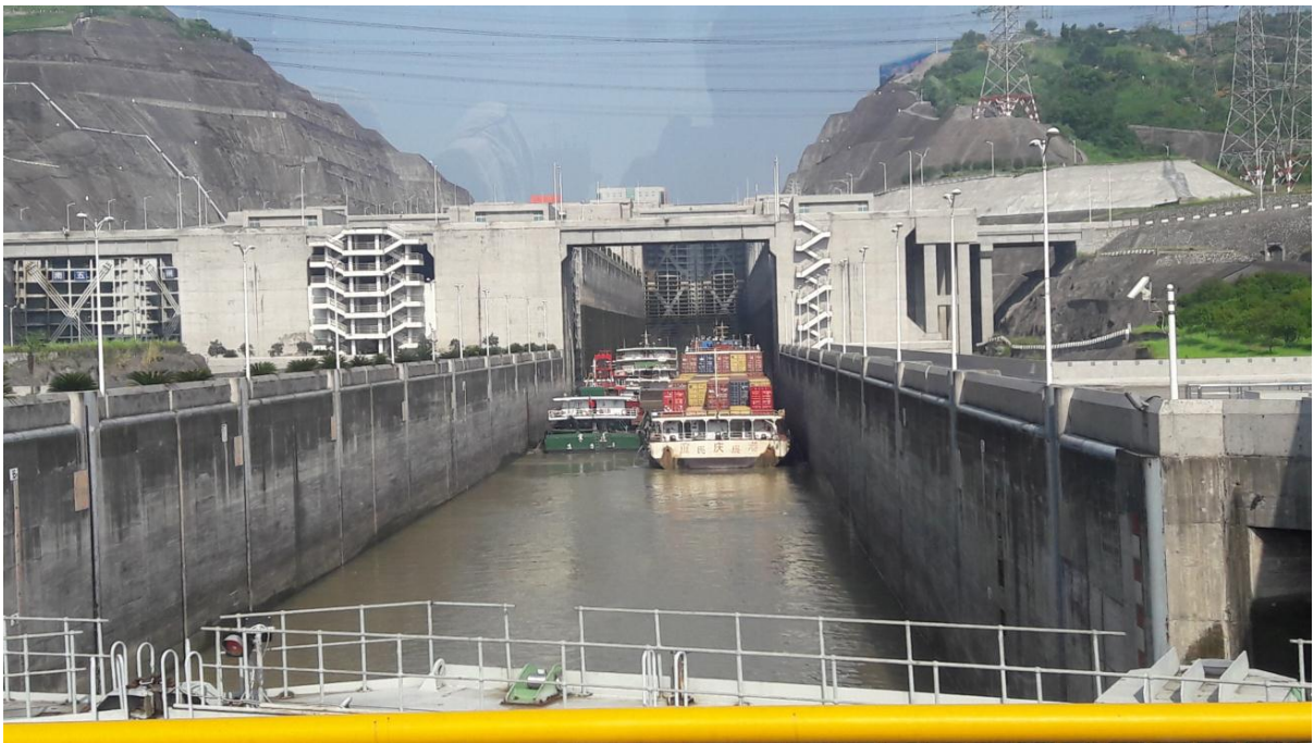
Figure 6 Navigation Locks at The Three Gorges Dam on Yangtze River
