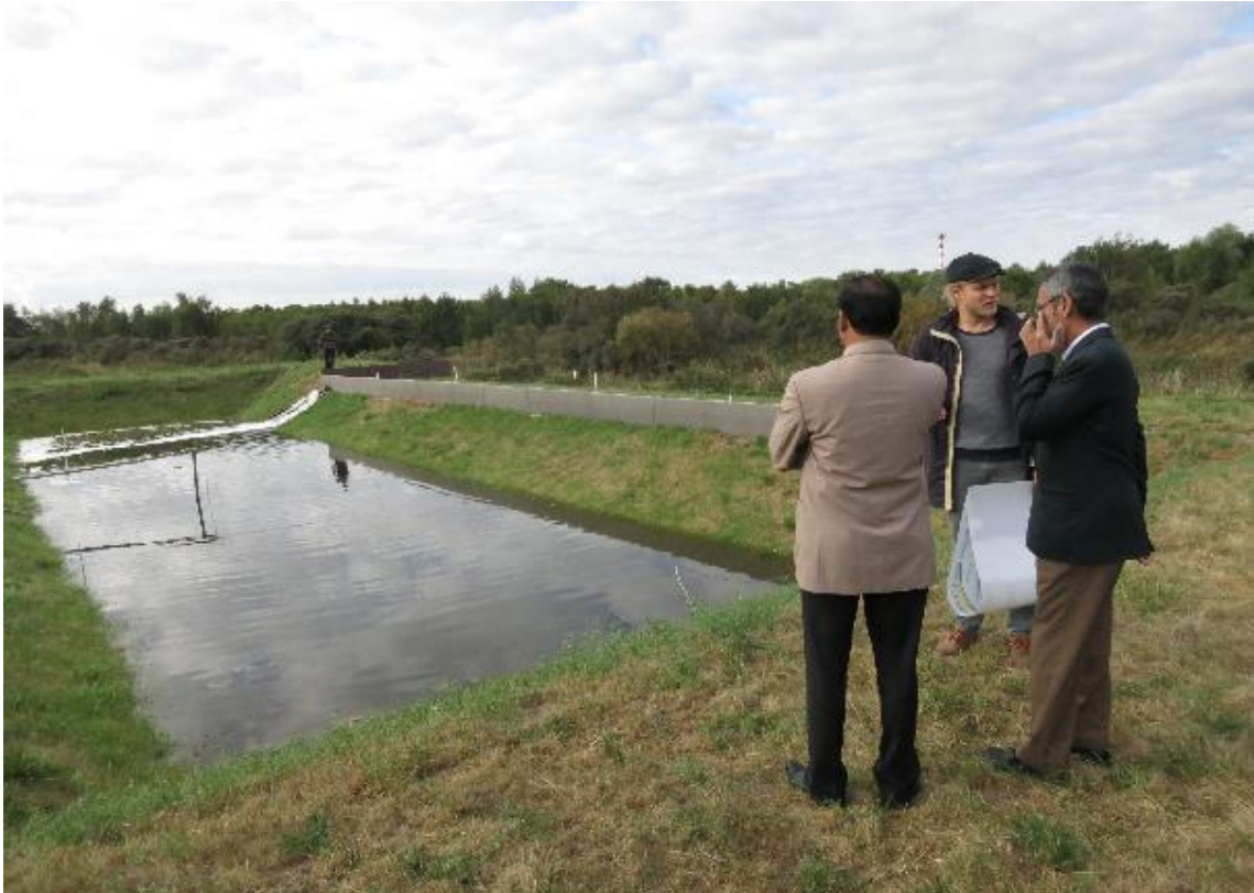
Figure 9. Test dikes with dredge fill material in Rostock
