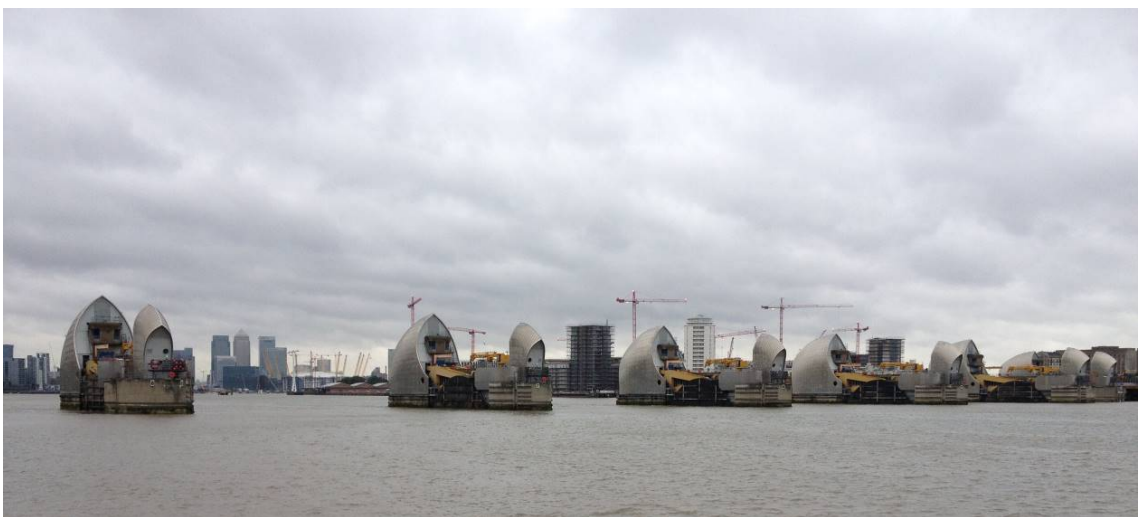
Figure 3. Thames barrage, 16 September 2016
