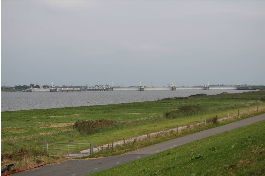
Figure 6. Ems barrier, about 500m long with two navigation openings (on the left hand side)
