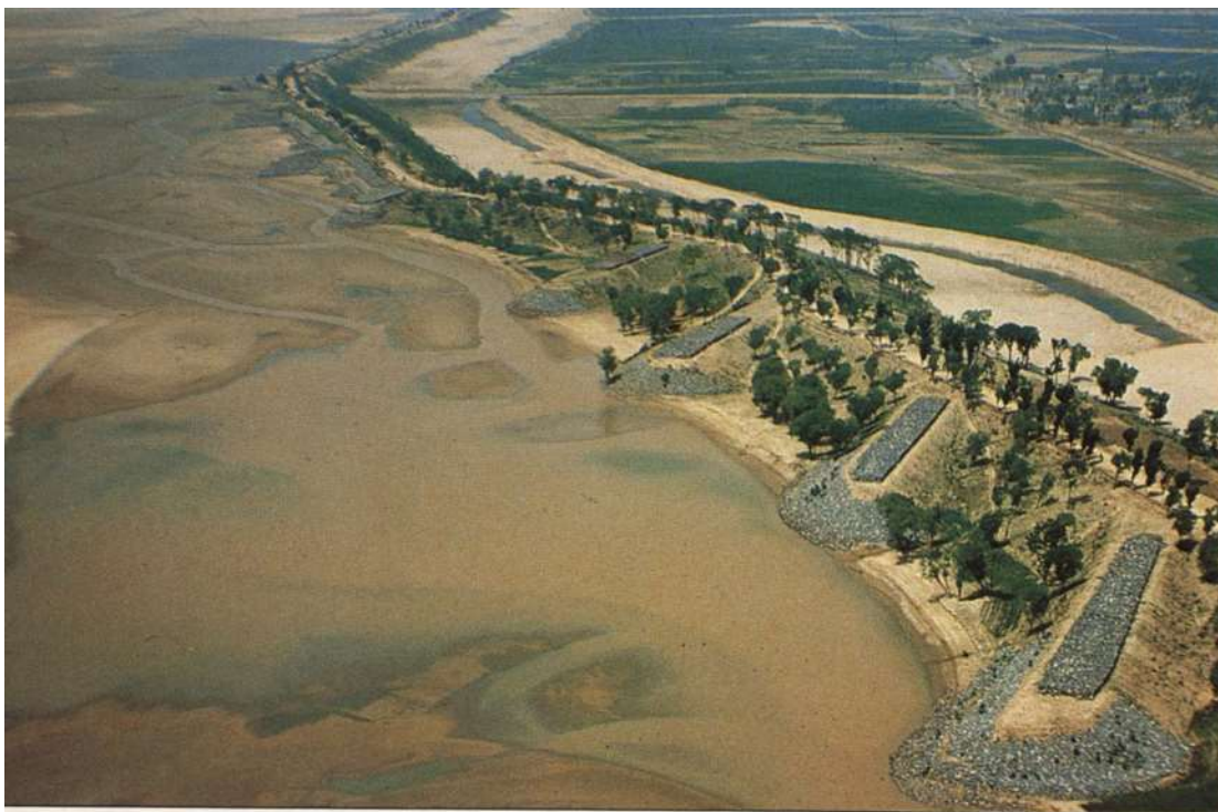
Figure 11 Spur dikes at Caogang in Henan Province
