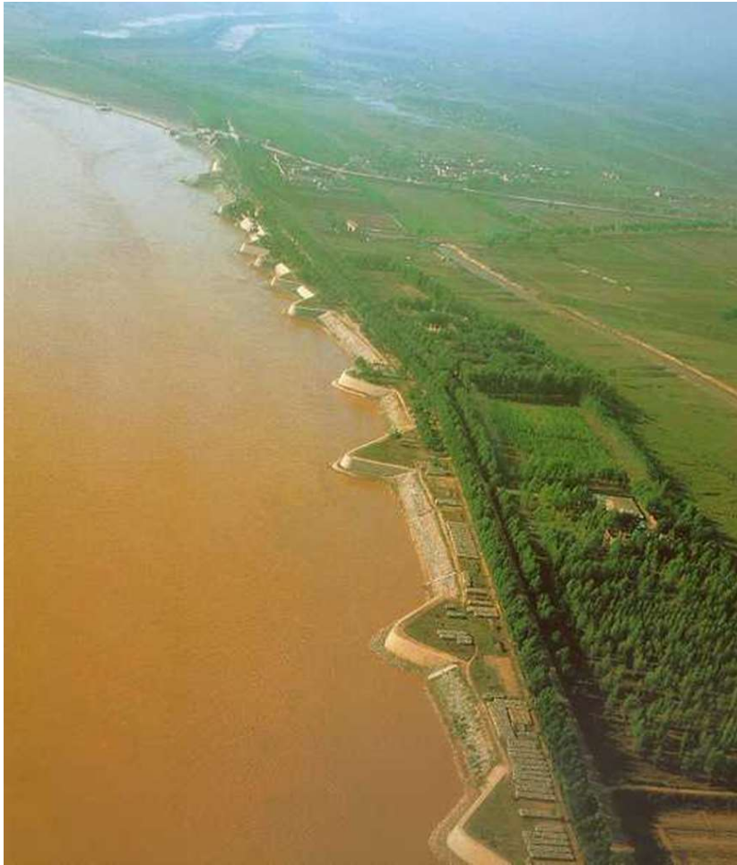
Figure 12 Spur dikes at Liuyuankou in Henan Province
