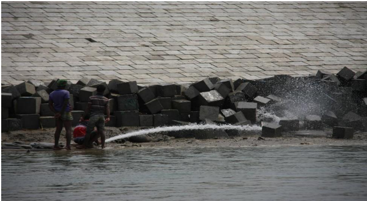
Chauhali correction of key level by removing earth deposit
