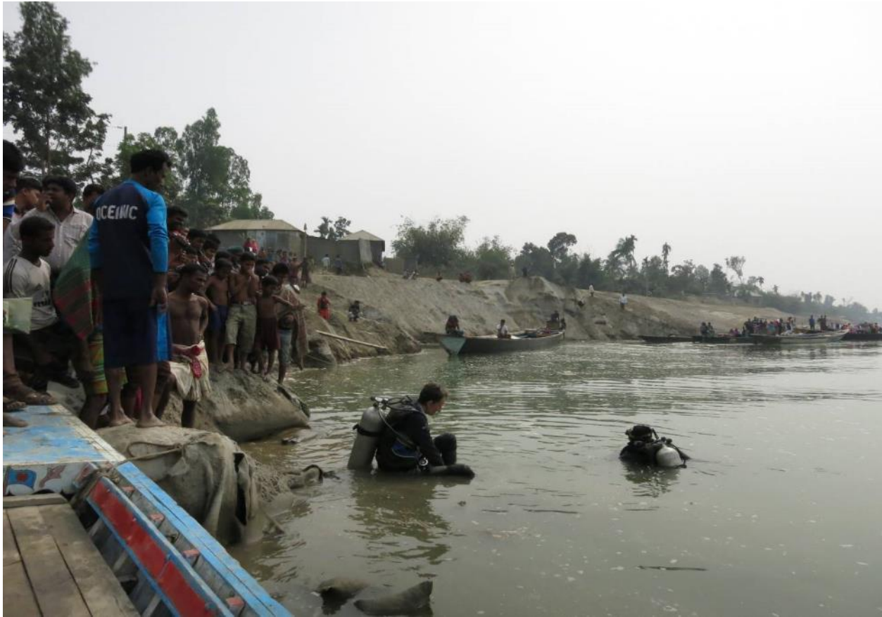
Chauhali diving investigation in geotechnical failure zone
