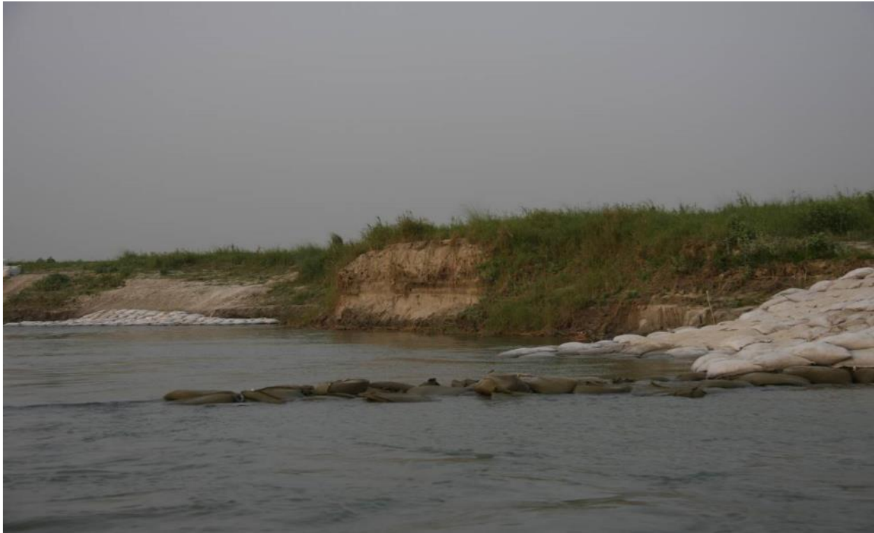
Harirampur Repair works on eroded wave protection (underwater protection in foreground)
