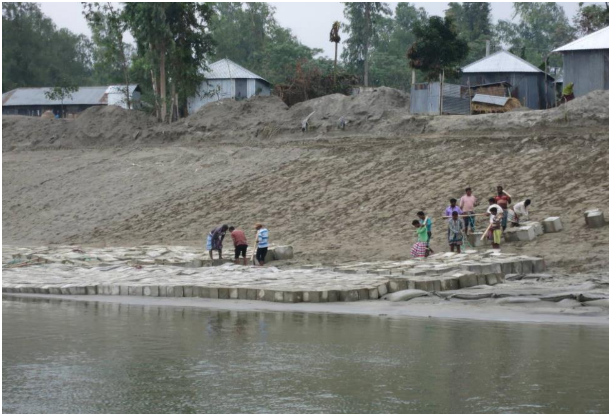
Chauhali concrete block key alternative placement for better access to the river
