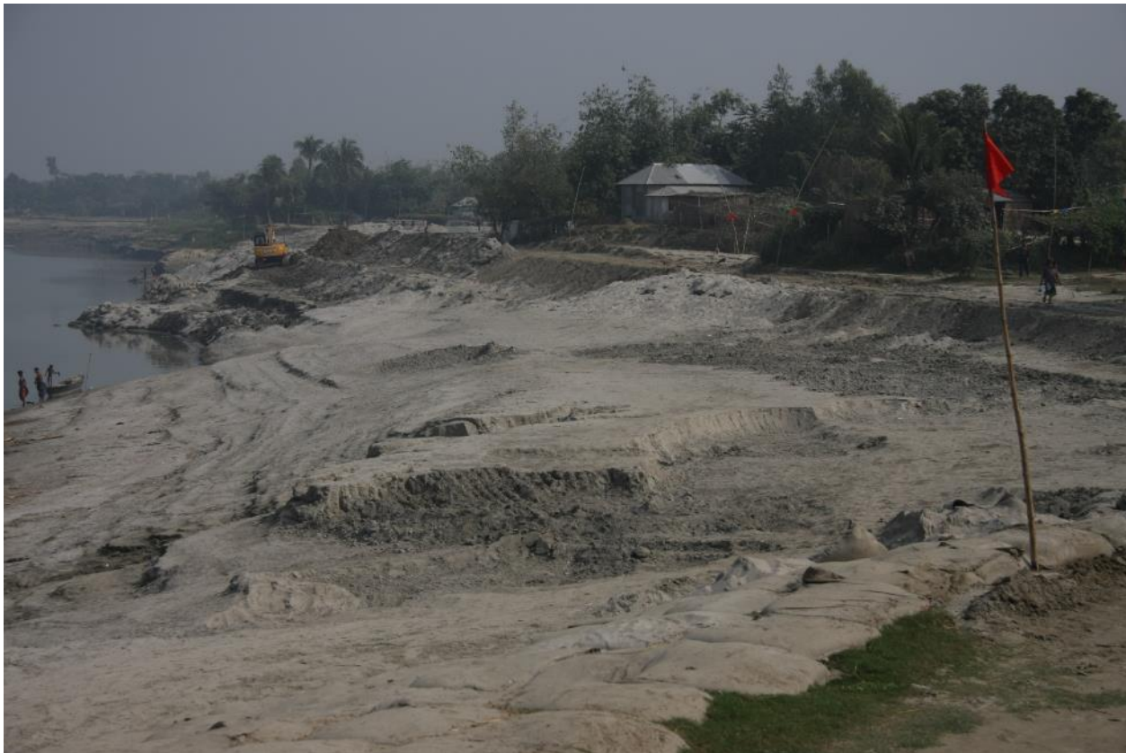
Zaffarganj commencement of excavation for the placement of permanent wave protection
