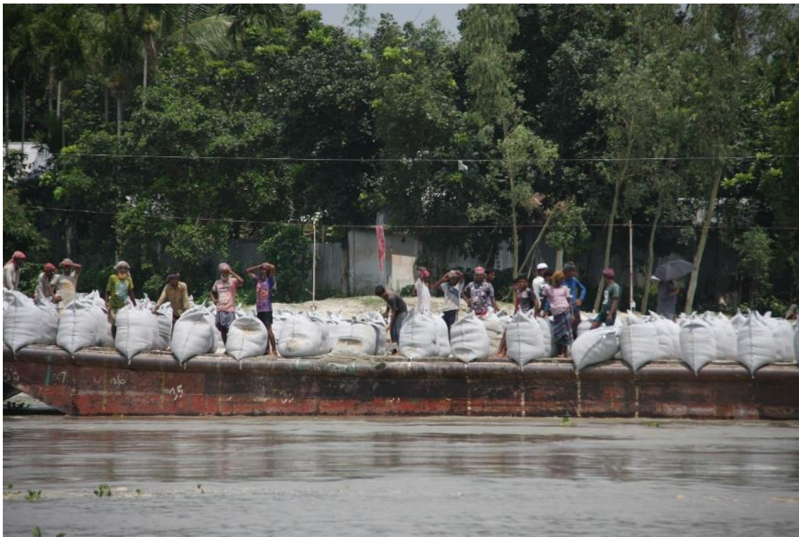
Chauhali: ongoing repair works in areas with slope failure, 10 June 2017
