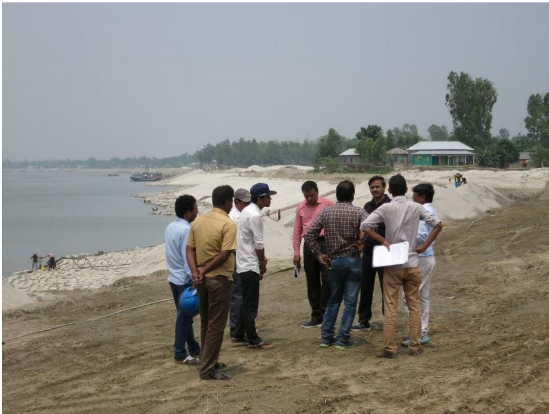
Chauhali: site visit of Project Director, 4 April 2017
