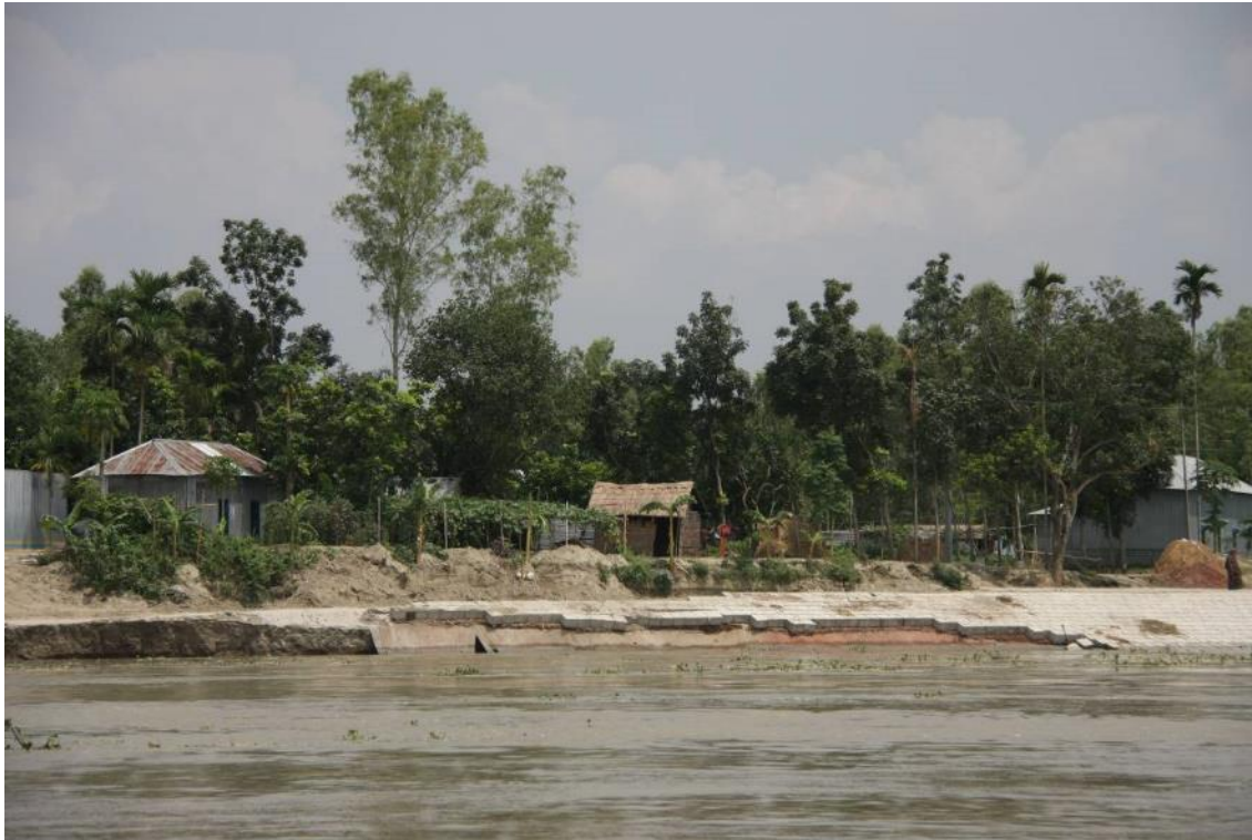
Chauhali: local failure of upper slope, 10 June 2017
