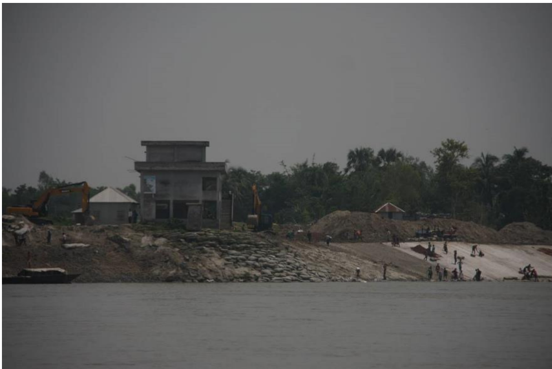
Zaffarganj: work around the old school building to be dismantled, 1 May 2017
