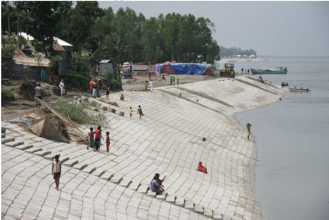
Chauhali: completed revetment between bridge and contractors camp, 1 May 2017
