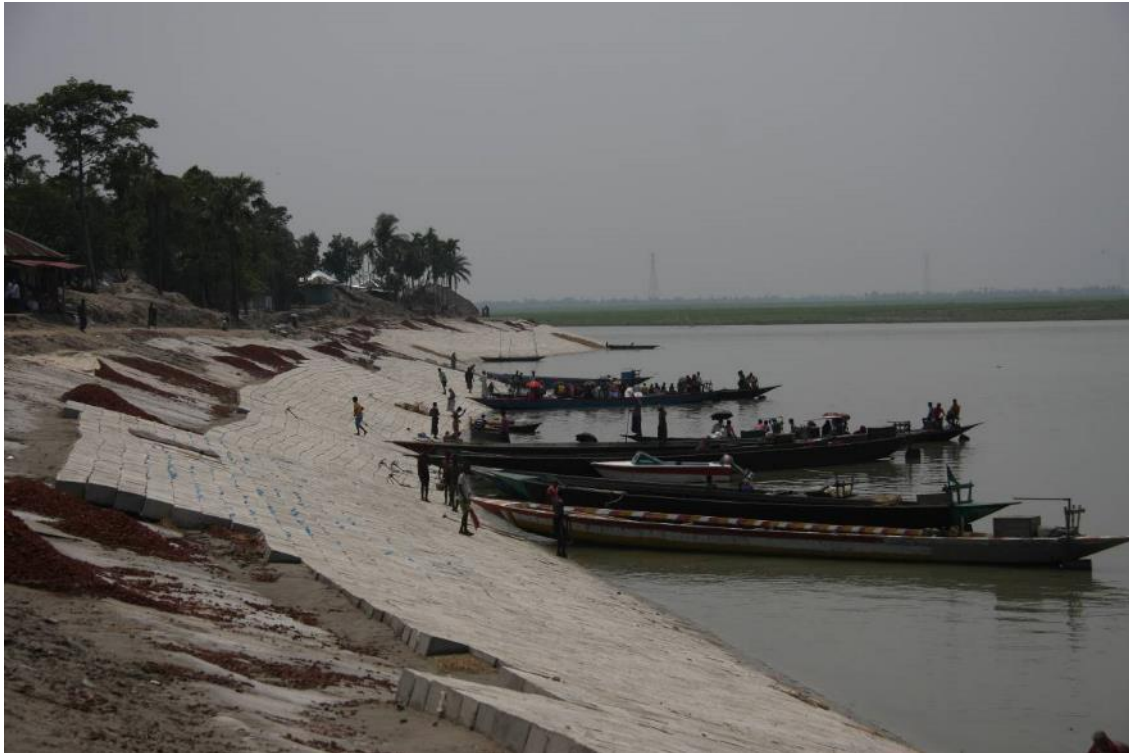
Zaffarganj: construction of final wave protection, 1 May 2017
