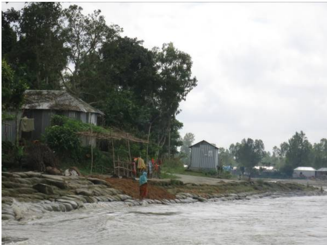
Photo 3. Chauhali upstream temporary wave protection of 2km length without damages, 1 Oct 2017
