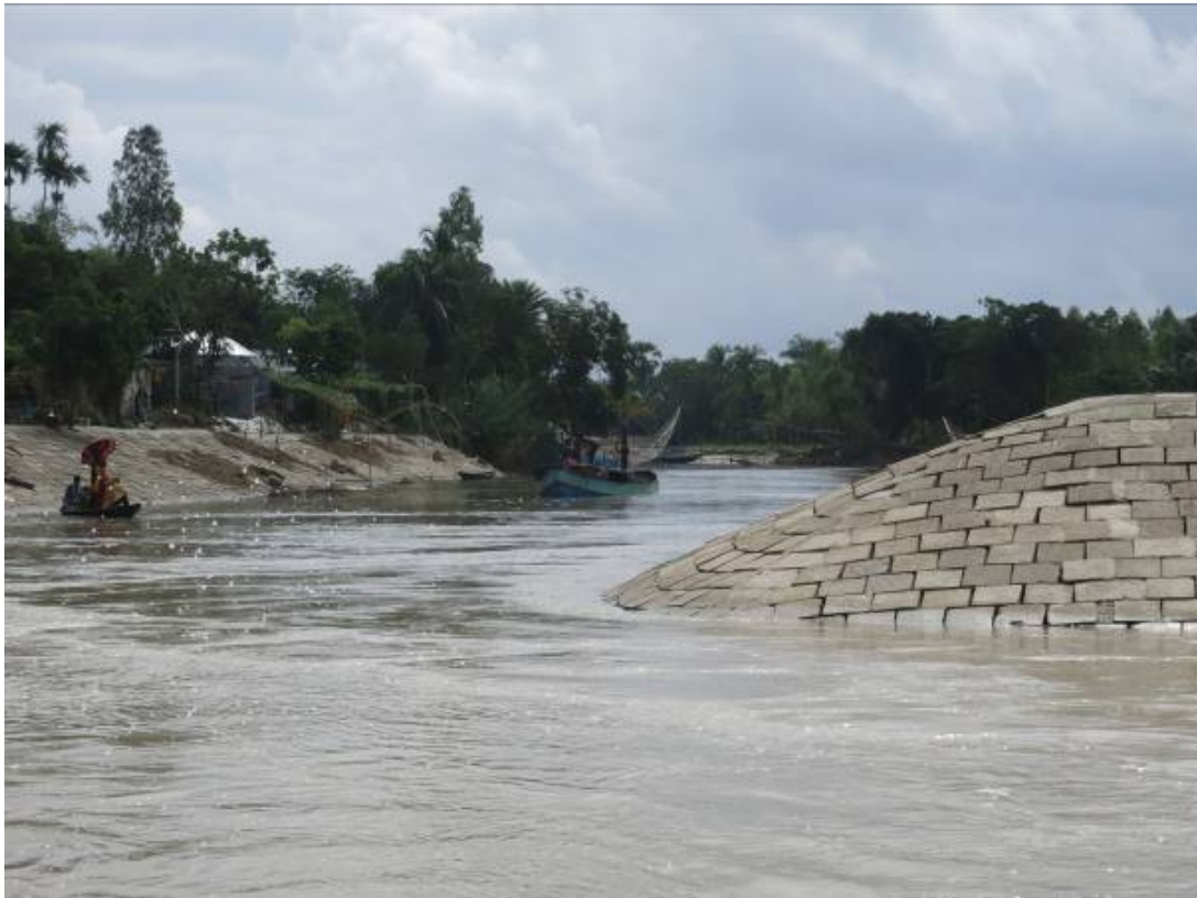
Photo 8. Upstream termination of Zafarganj work with offtake channel protection, 1 Oct 2017
