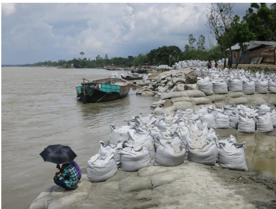
Photo 6. Solimabad, ongoing emergency works, 1 Oct 2017
