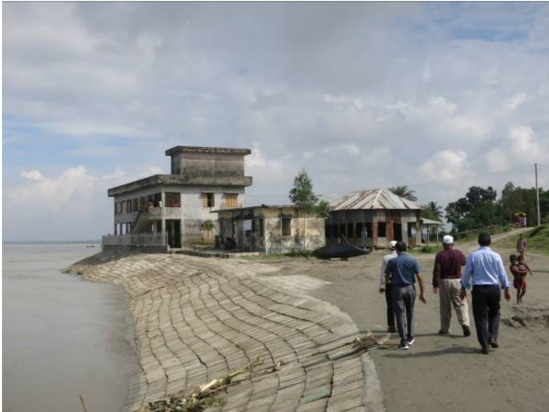
Photo 7. Visit of temporarily protected school at Zafarganj by Chief Planning, Chief Monitoring and Chief Engineer Design, 1 Oct 2017
