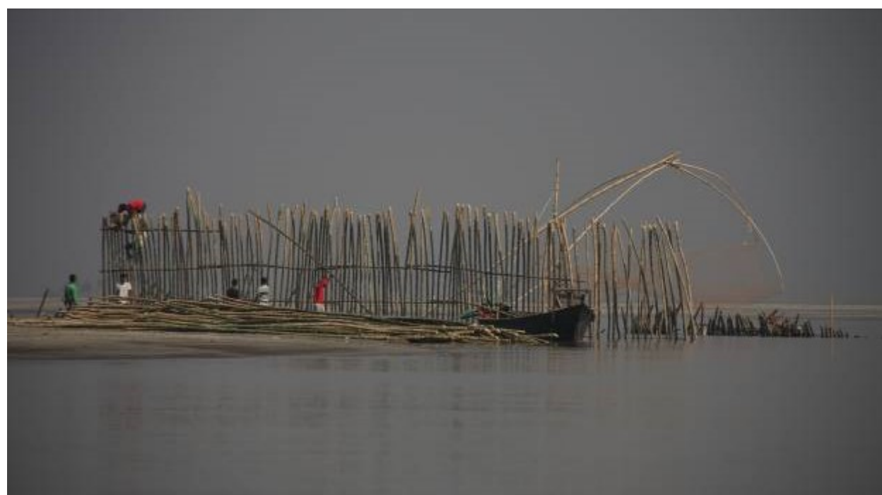
Photo 6. Bandalling erosion protection 8 works along Kojjuri revetment, 1 December 2017
