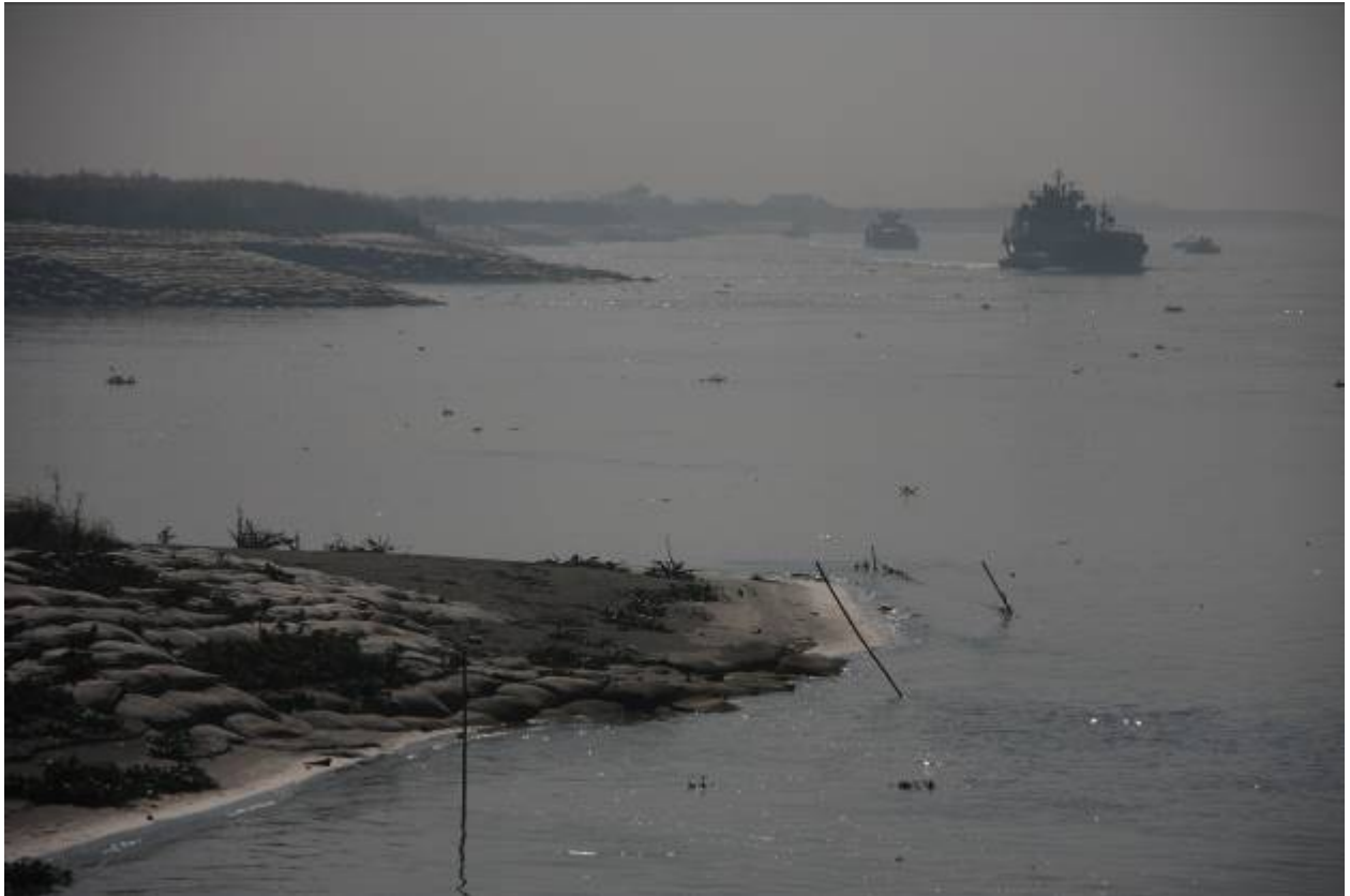
Photo 11. Revetment work alongside major navigation route at Harirampur, 12 December 2017
