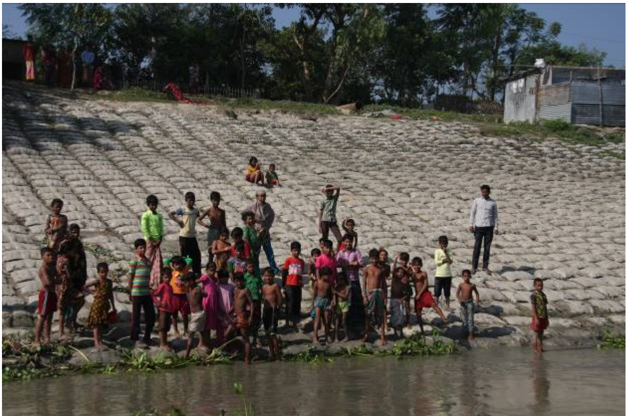
Photo 4. Grout-filled mattress installed in 2006 at Koitola, 1 December 2017
