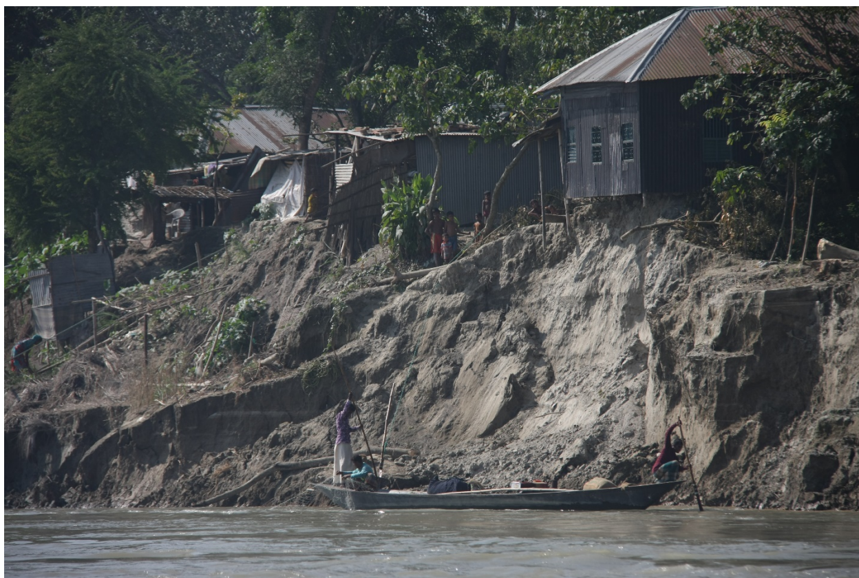
Photo 5. Riverbank erosion between Kojjuri revetment and Hurashagar, 1 December 2017
