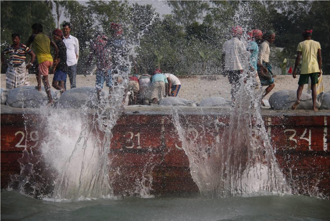
Adapatation work at Chauhali, last work from contract W06, 18 Feb 2018
