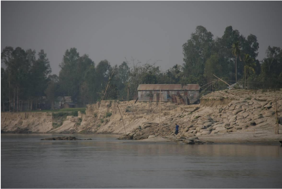
Erosion upstream of Chauhali, with beginning of outflanking of the existing works, 18 Feb 2018
