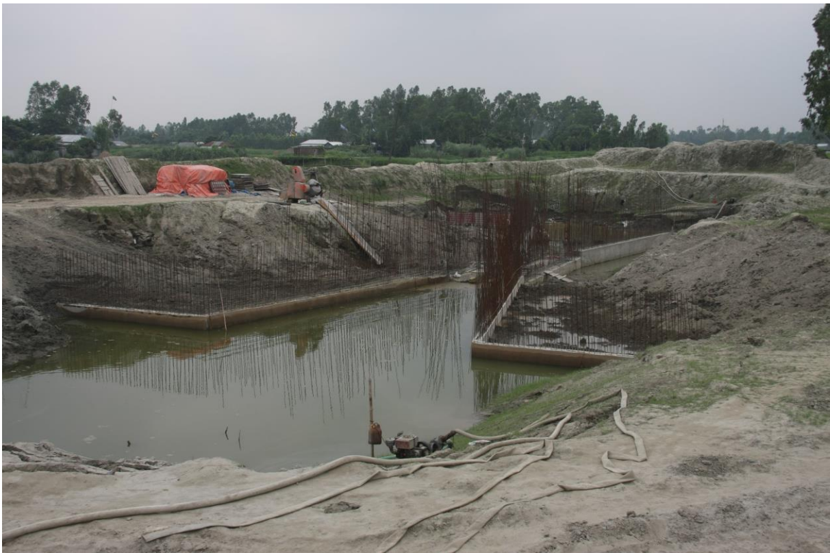
Construction of Kojjuri Regulator, Package W-01
