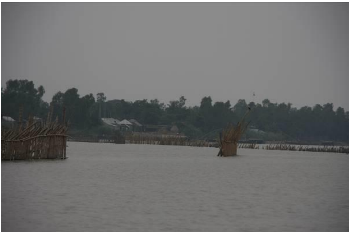
Bandalling at Benotia to counter riverbank erosion
