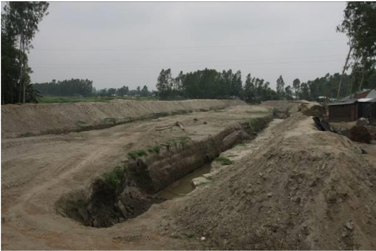
Preparation of embankment construction, contract package 3
