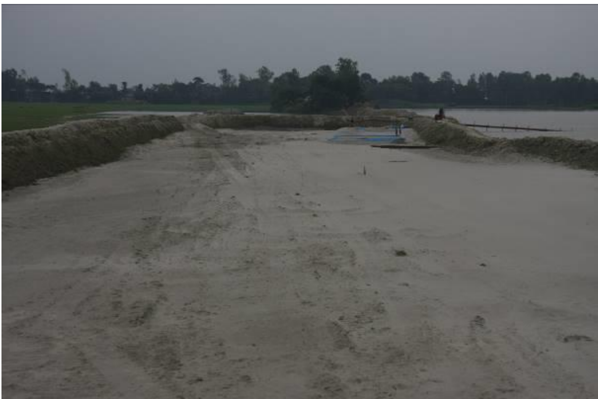
New embankment construction alongside the Hurashagar River, contract package 4
