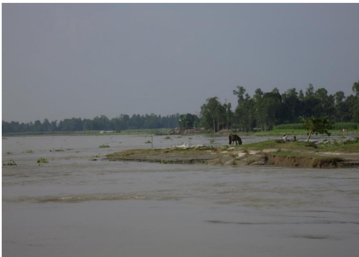
Chauhali, 23 September upstream outflanking erosion addressed by BWDB, Tangail Division
