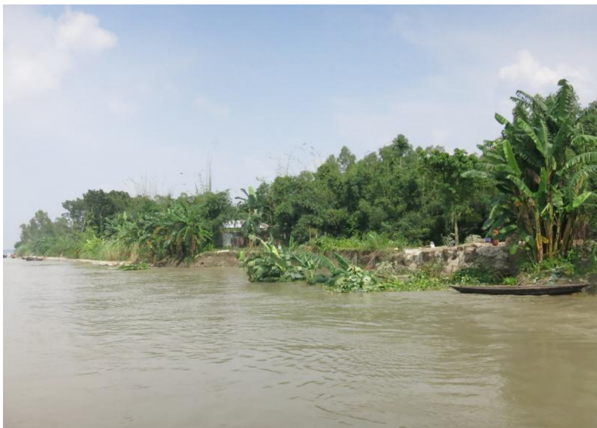
Chauhali, 23 September, downstream failure
