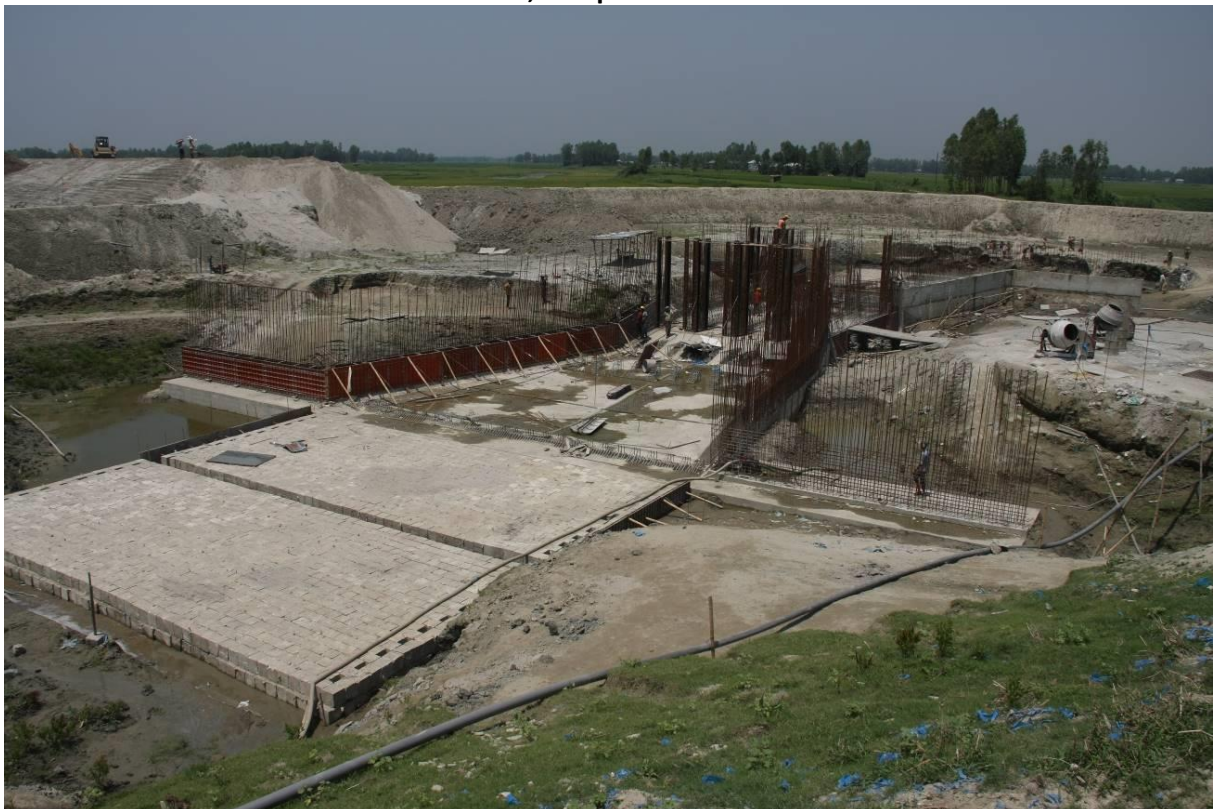
Figure K8: Harirampur embankment, regulator construction package 4, 20 April 2019
