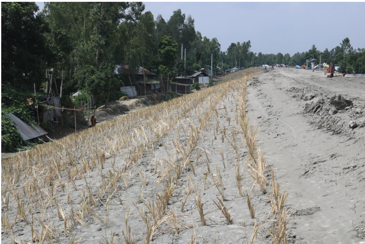
Figure K11 : PIRDP, revetment protection constructed between 2004 and 2006, maintenance free performance
