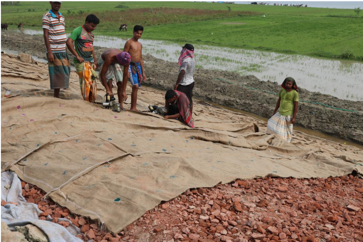
Figure K 14 :Slope preparation in grout filled jute mattress works
