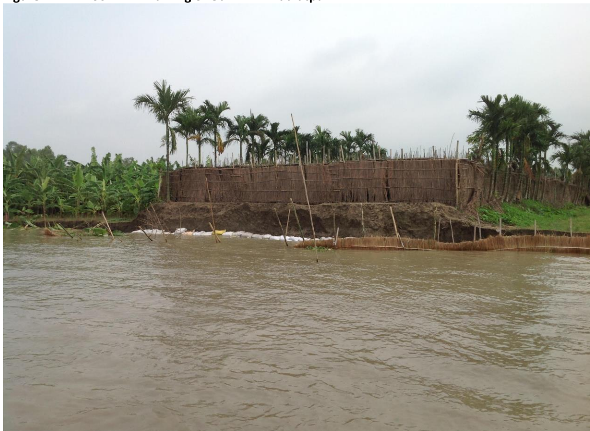
Figure K 18 : 2019 Flood situation in Harirampur ( July 2019)
