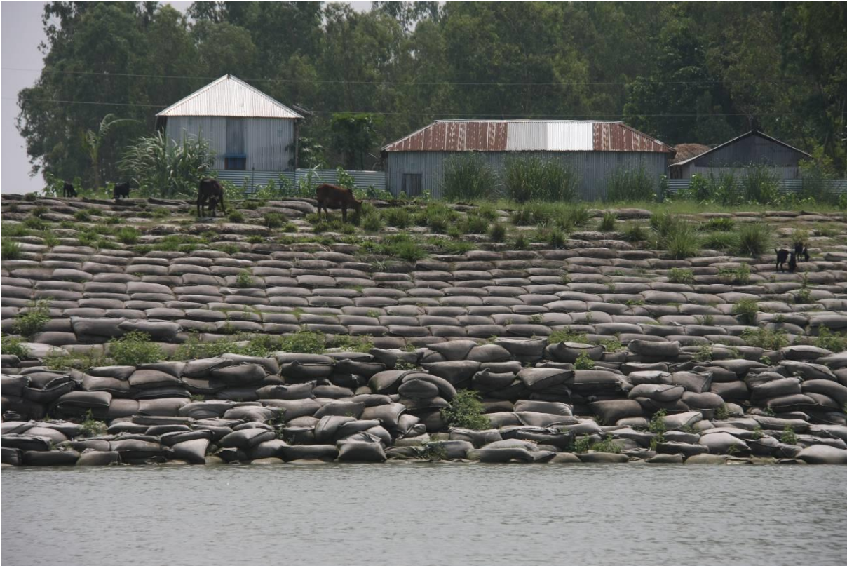
Figure K5 :Chauhali, temporary wave protection between km 5 and 7 intact after 3 years, 20 April 2019
