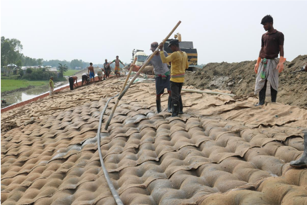
Figure K13 : Concrete pumping in grout filled jute mattress works
