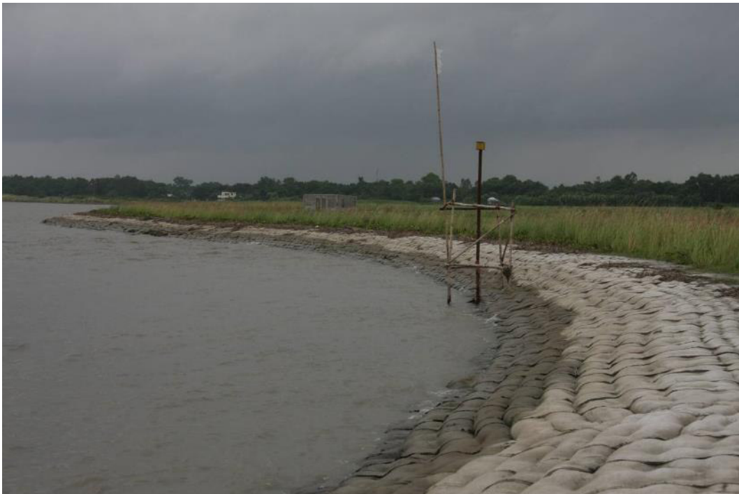
Figure L-12 Harirampur grout filled mattress with vetiver plantation and measurement station, 13 Sep 2019
