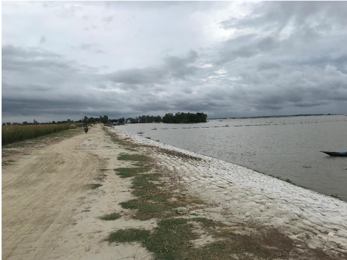
Figure L-5: W14 Pilot work site at Bera embankment, 24 Sep 2019
