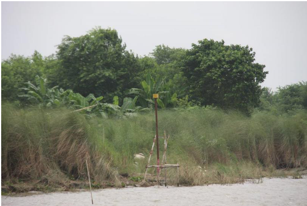
Figure L-14 Harirampur geobag protection with plant cover and downstream measurement station, 13 Sep 2019
