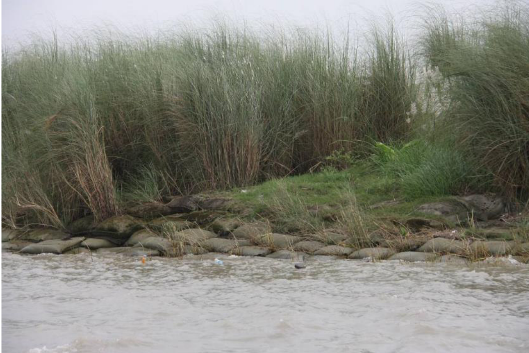
Figure L-15 Harirampur geobag protection with plant cover, 13 Sep 2019
