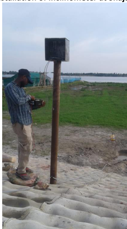
Figure L-18 Installation of piezometer at Shajadpur, 29 Aug 2019
