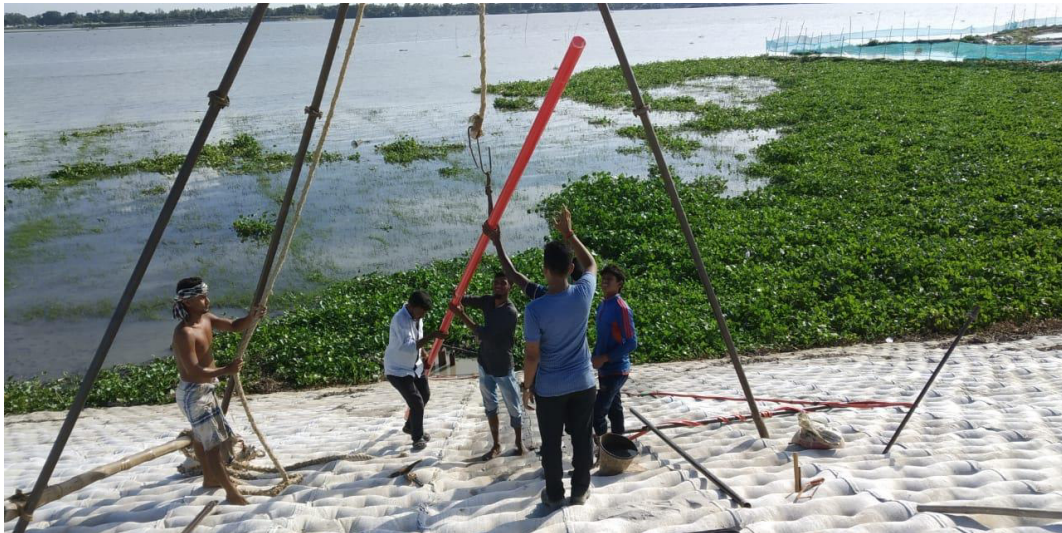
Figure L-16 Installation of inclinometer at Shajadpur, 29 Aug 2019
