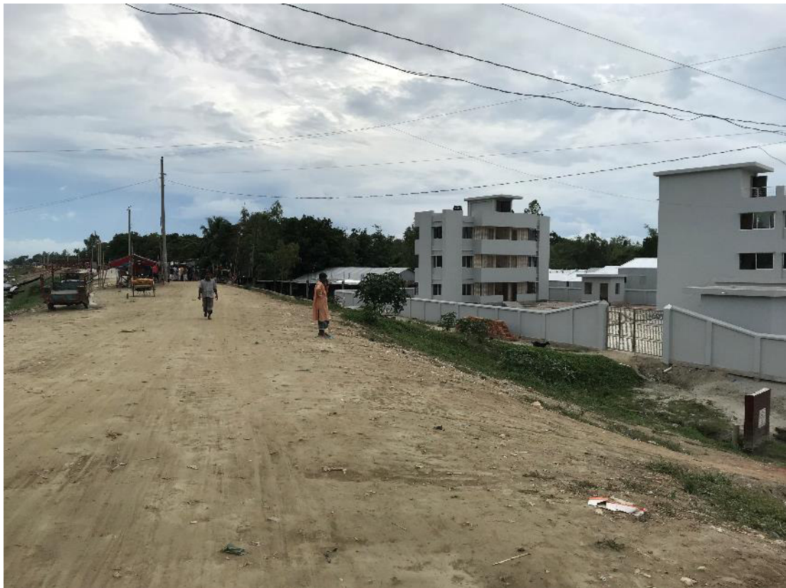
Figure L-6: A new hospital and a growth center located behind the new embankment, 24 Sep 2019
