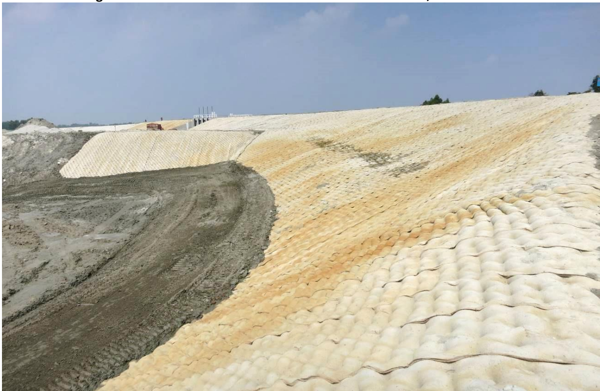
Figure L 8: Dutch Ambassador visits FRERMIP, grout-filled juste mattress works at Kaijuri, 6 March 2020
