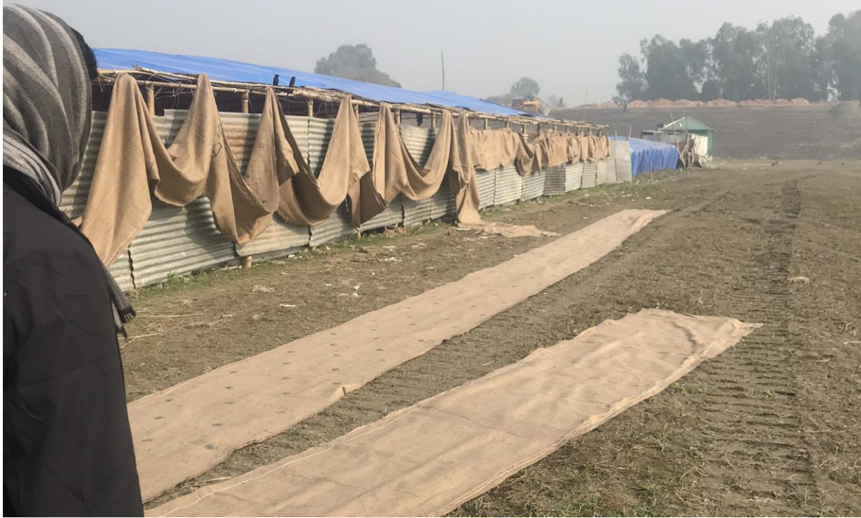
Figure L 11: Jute fabrication for grout filled mattress at Sahzadpur, W16 package
