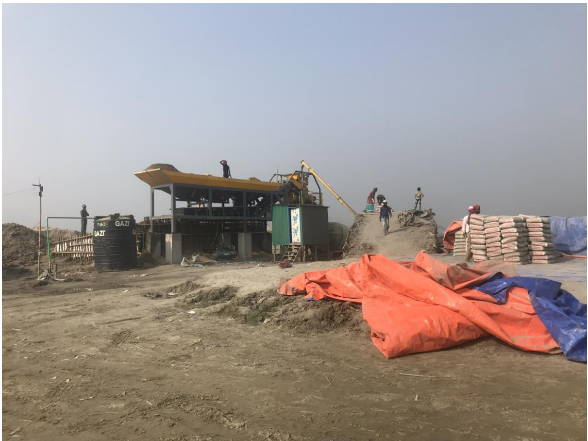
Figure L 12: Jute fabrication for grout filled mattress at Sahzadpur, W16 package
