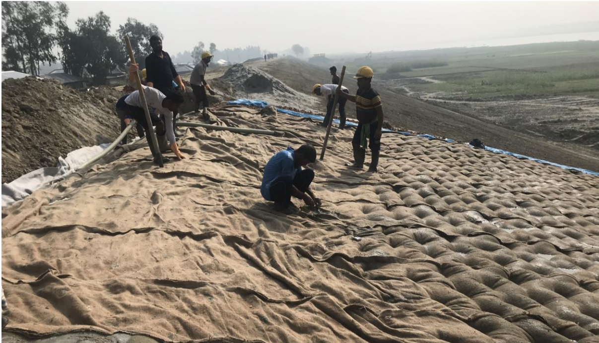
Figure L 14: Grout filling, W16 package
