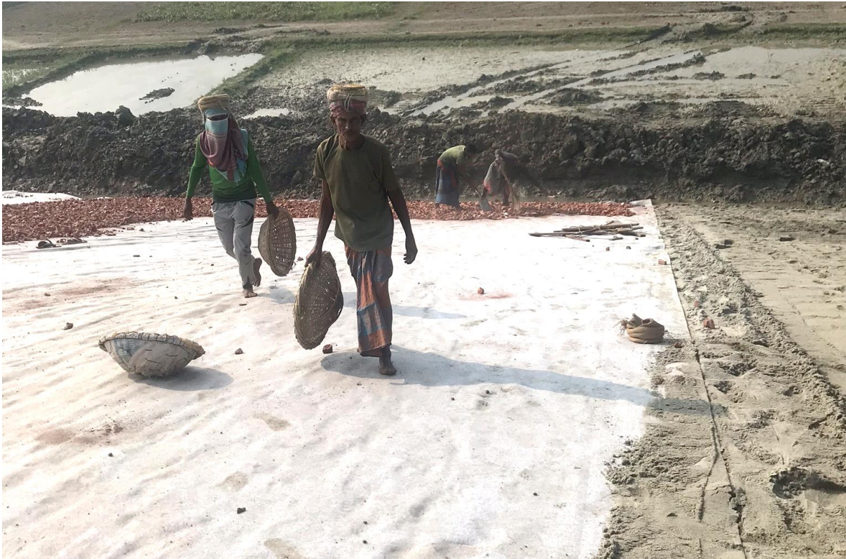
Figure L 13: Slope preparation for Grout filled mattress, W16 package
