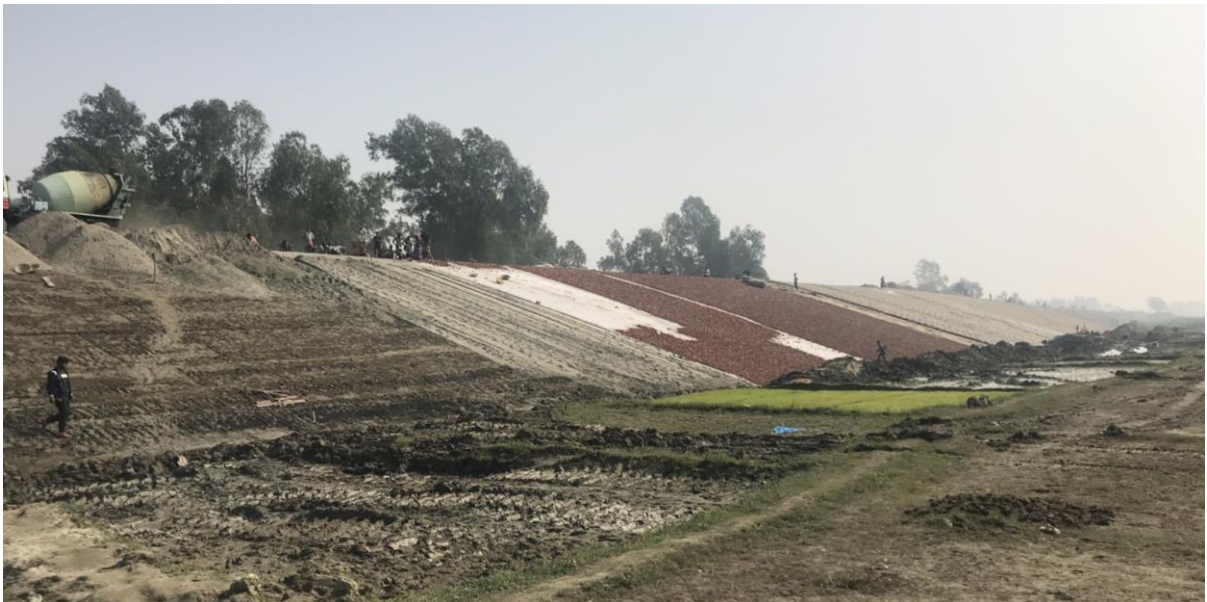
Figure L 14: Slope preparation for Grout filled mattress, W16 package
