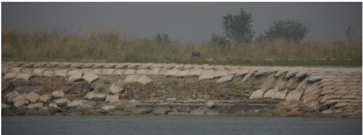
Figure 3-17 Schematic of slope erosion due to under-designed temporary wave protection
