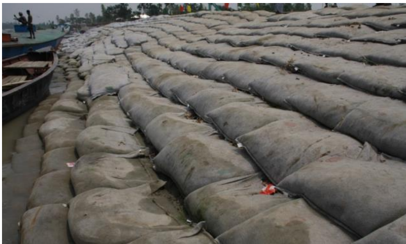
Figure 3-11 Temporary slope protection consisting of one layer of geobags
