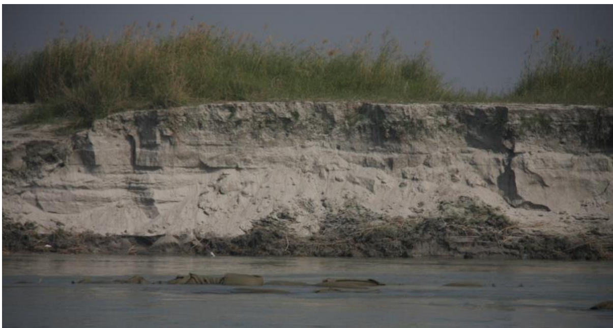
Figure 3-18 Progression of destruction of temporary slope protection: (1) surface protection disintegrates into elements (through high velocities or wave impact) (2) hole eroded in bankline with regressive erosion and deepens, but underwater protection is still in place (foreground at low water level)
