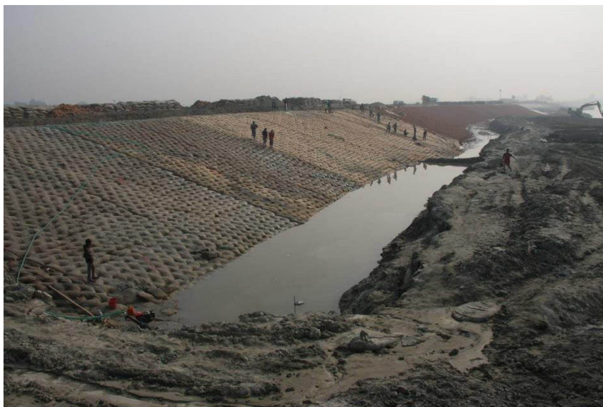
Figure 4-3. Installation of grout-filled jute mattress (Harirampur Feb 2019)
