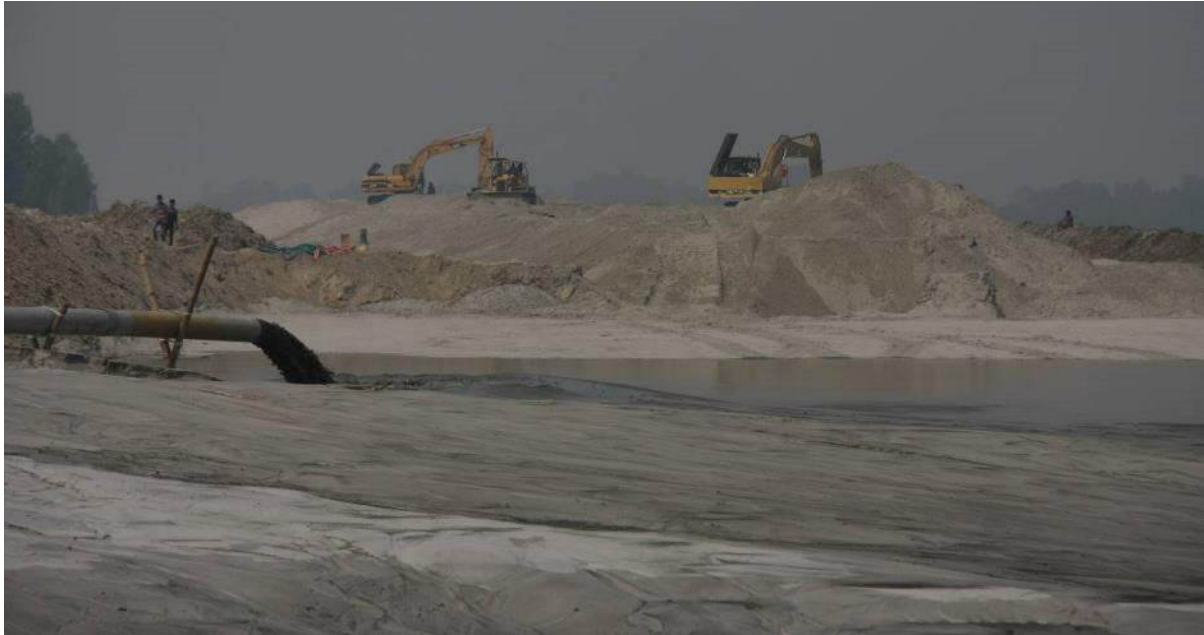
Figure 4-4. Embankment construction at JRB-1 with compacted dredged sand (Kaijuri, Feb 2019)
